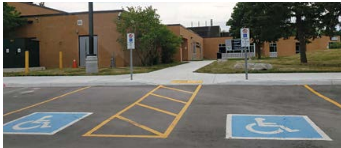
Accessible parking markings and accurate signage
